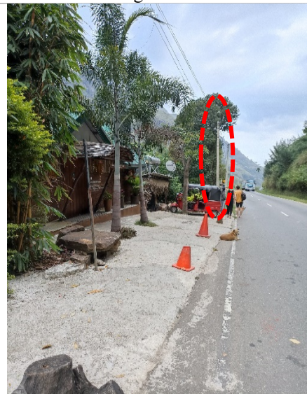
Figure 6d: Electricity line
