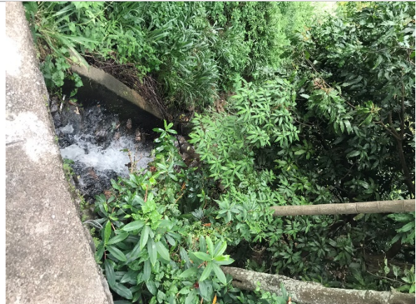
The drainage running in the downslope
