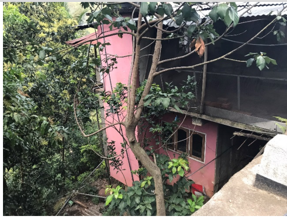
Commercial building located in the down slope
